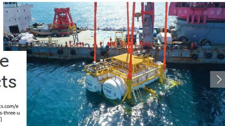
...le of the Hainan Undersea Data Center is launched on March 31 in Lingshui Li autonomous county of Hainan province.
